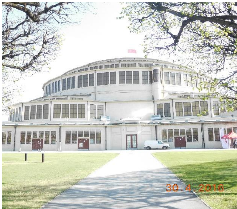
Built 1912/1913, the “Centennial Hall” in the European Capital of Culture Wrocław/Breslau, named after an exhibition that was organized in 1913 to commemorate the liberation of Germany from Napoleon 100 years ago. It is a UNESCO World Heritage Site.
