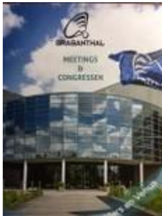
Versatile, comfortable conference facility on the outskirts of the University city of Leuven (BE)
